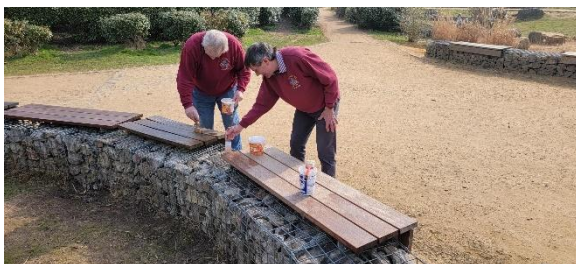
Special Projects Group varnishing newly installed benches
