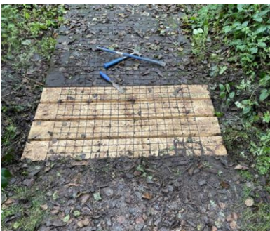
Ongoing board walk repairs in BI
